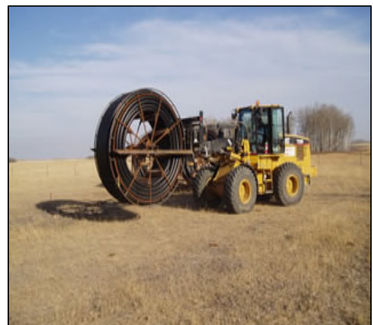
Coiled pipe is quicker and easier to install
