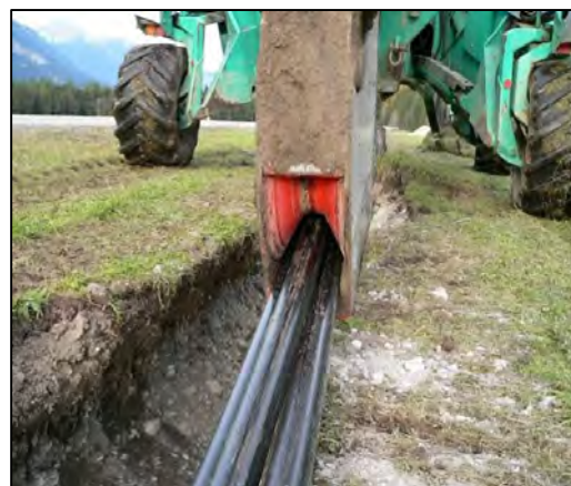
Trenching laying multiple lines
